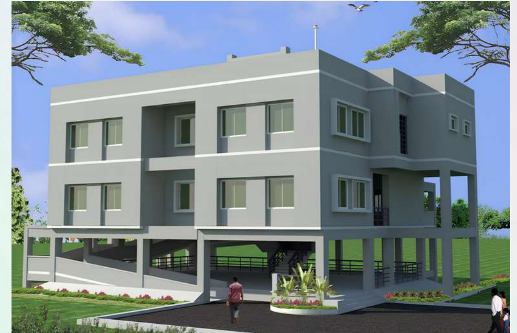
100 CYCLONE SHELTERS MINISTRY OF DISASTER MANAGEMENT & RELIEF
